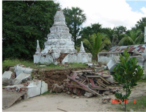
Fig.22.Photo shows damage of pagoda in Taungdwingyi by 2003 earthquake (Source:MEC)
