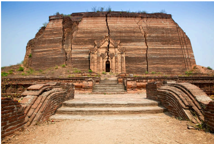
Fig.19. The Mingun Pagoda the world's largest brick stupa was damaged by the 1839 Ava earthquake and the 1956 Sagaing earthquake.
