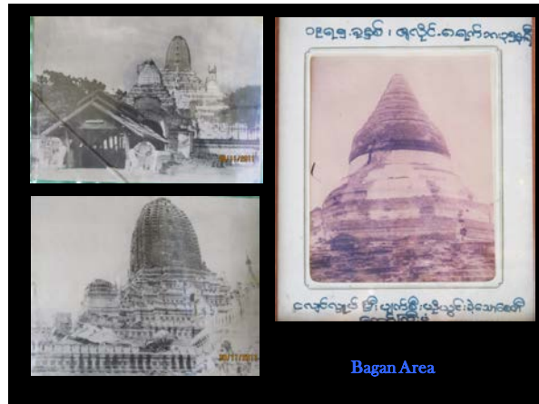
Fig. 20. Damage of pagodas by the 1975 Pagan earthquake (Lin Thu Aung)
