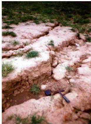
Fig.23.Photo shows ground failure in Taungdwingyi
